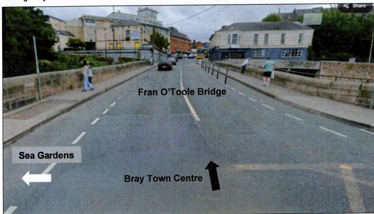
Figure 5-1: Existing Fran O'Toole Bridge with Footpaths and Cycle Lanes
